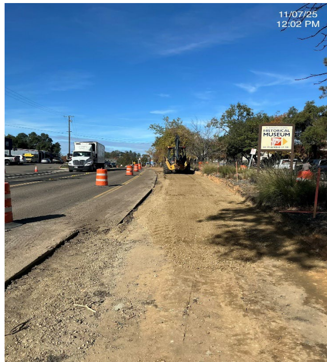
Demolition and Subgrade Prep on East Side
