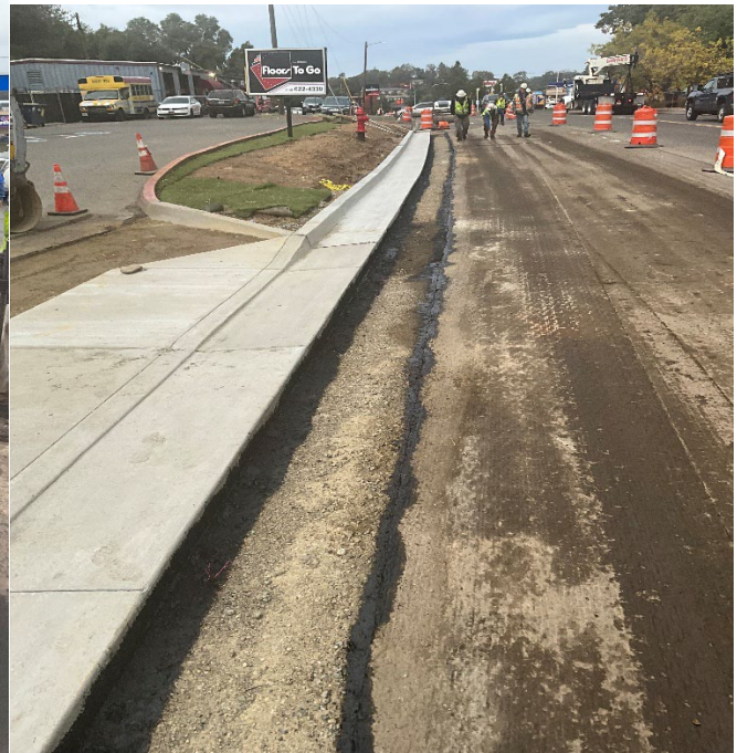
Demolition and Subgrade Prep on East Side
